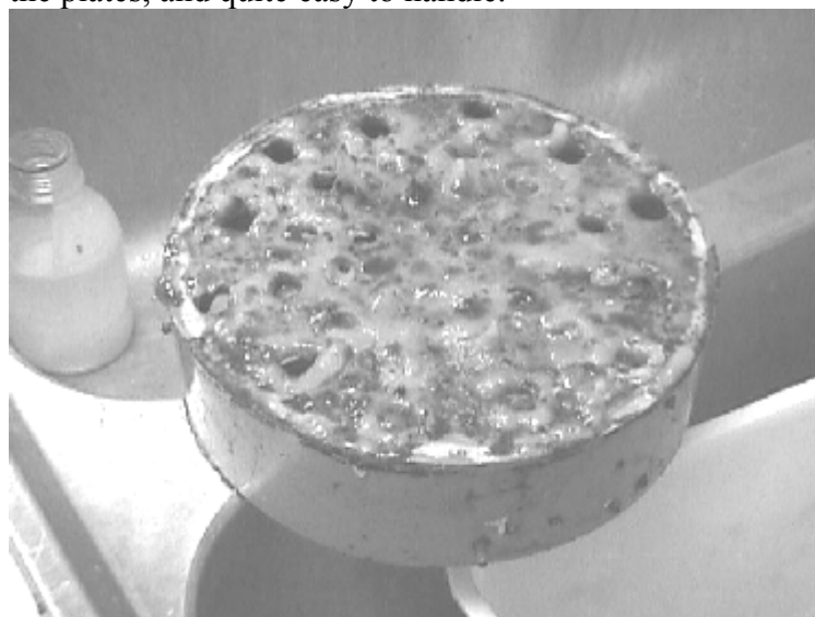
Figure 1 Liquid distributor showing the growth of biomass on the lower surface. The same occurrence, even stronger, could be observed on the top side.
